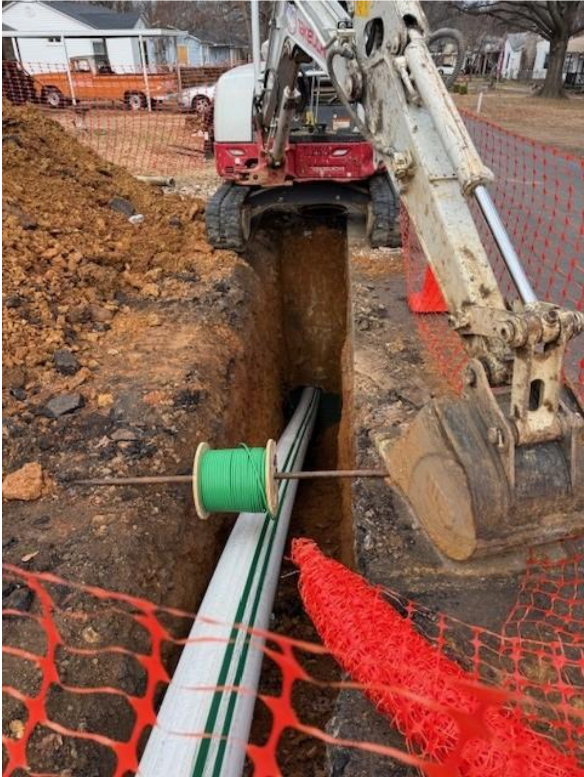
Sending Pit for HDPE Pipe Bursting
