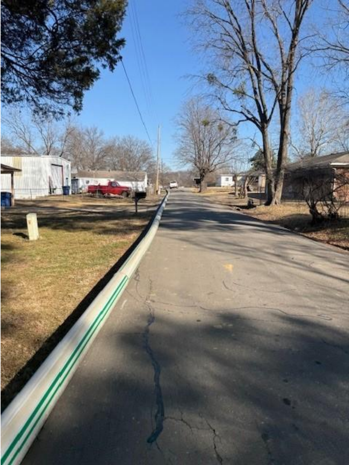
Fused HDPE laid out prior to installation
