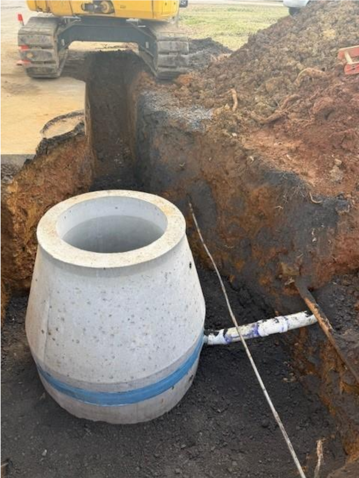
New Manhole with Sanitary Sewer Service
